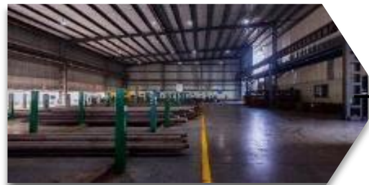
Covered Raw Material Yard
